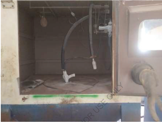
Fig 3.5: Grit blasting process
